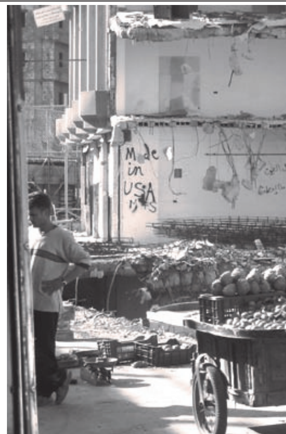
Bomb damaged home in south Lebanon with graffiti, “Made in USA.” (Photo by Susan Galleymore)
