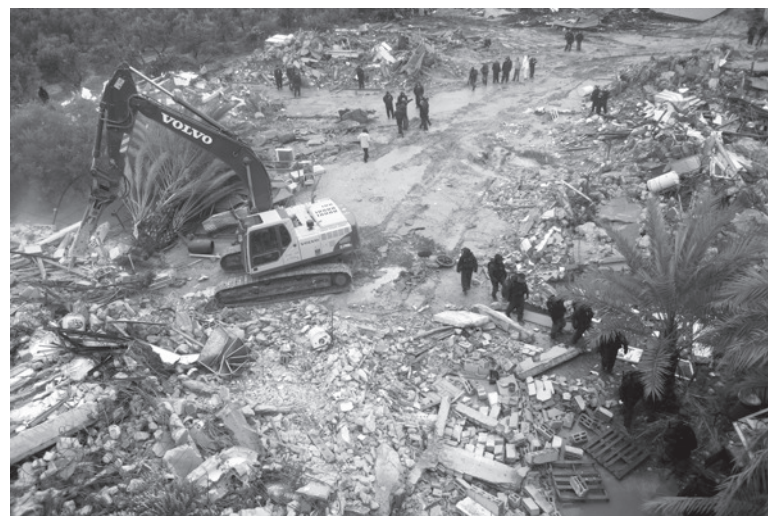
Israeli Riot Police guard a bulldozer during a house demolition. In Lod, Israeli authorities demolished the homes of seven Arab families in one day. (Photo credit: Oren Ziv/Activestills – see box below)
