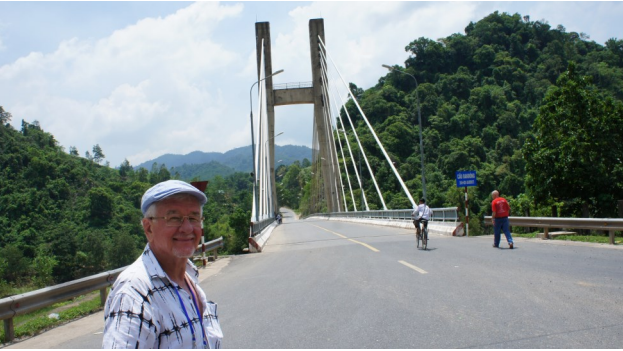
Da Krong Bridge, leading from Khe San to A Luoi, built for Viet Nam by the Cubans after the war, twice.
